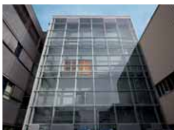
› A part of the building for the 300-millimeter pilot line in Villach (Austria)
